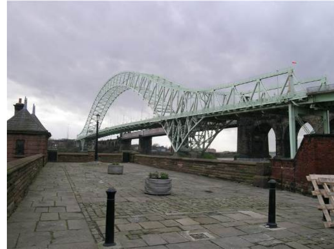
Existing Silver Jubilee Bridge
